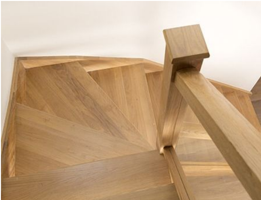
Fig -1 fitting a top or bottom winder
