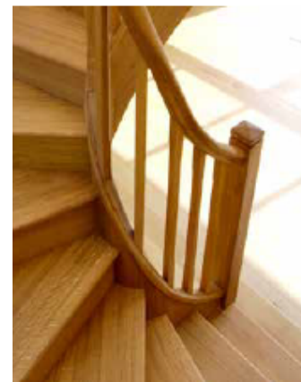
Fig -2 Handrails and balustrades
